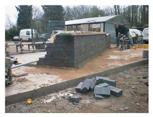
A variety of panels were built, and a range of materials used. Above we have one of the corner panels in engineering brickwork.
